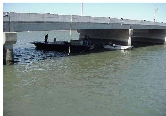
Bridge, Stone Harbor, New Jersey
