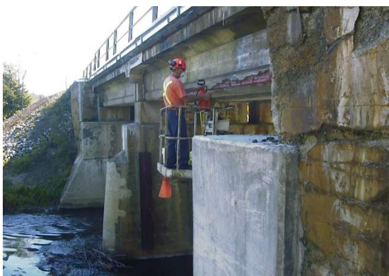
Bridge Chelmsford, Ontario
